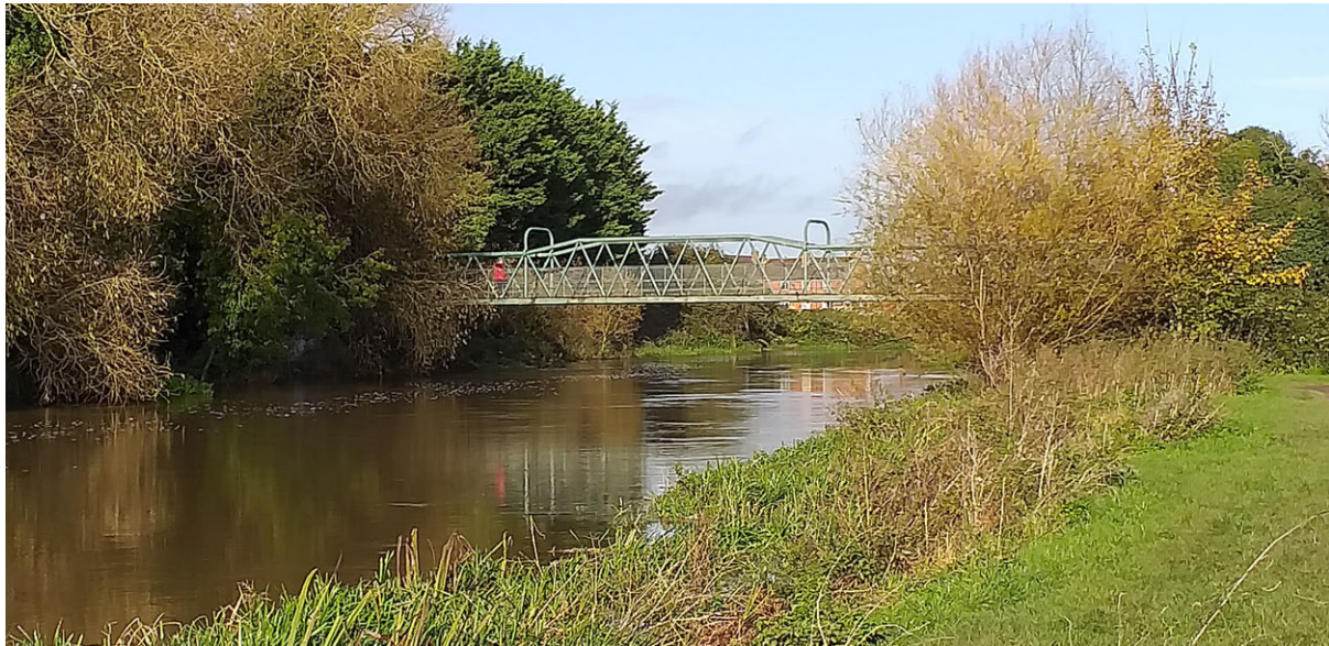
Photo 2A below – Looking north from Riverside Walk
