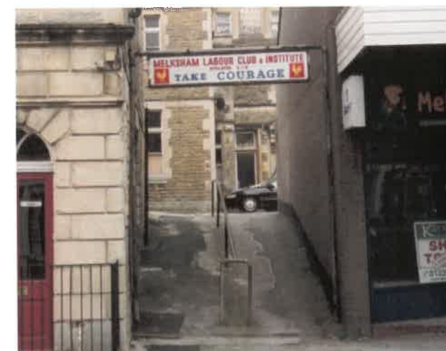
The entrance to the Labour Club is functional but lacks design and materials that are fitting for a central location on Bank Street. Project 35
