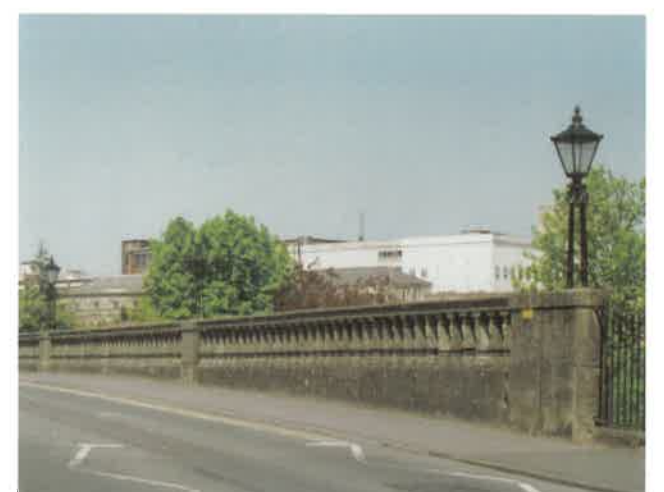
View over Avon Bridge
