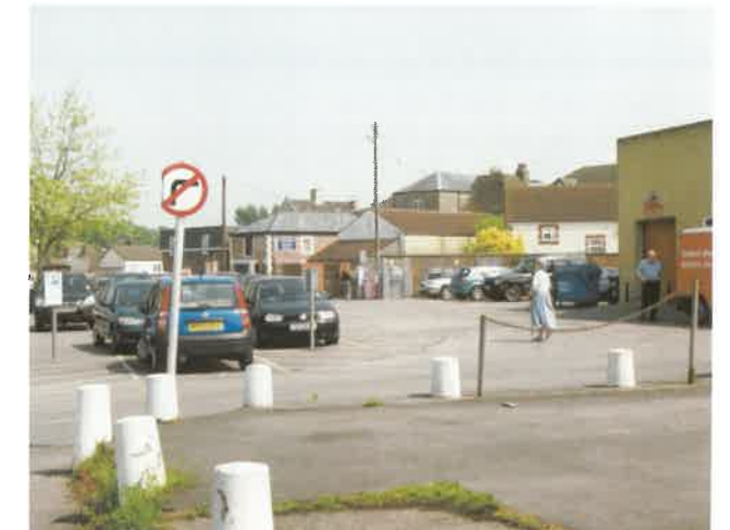
Church Street car park is a large characterless open space. Designing the car park as a space with improved legibility for pedestrians would enhance the important central area
