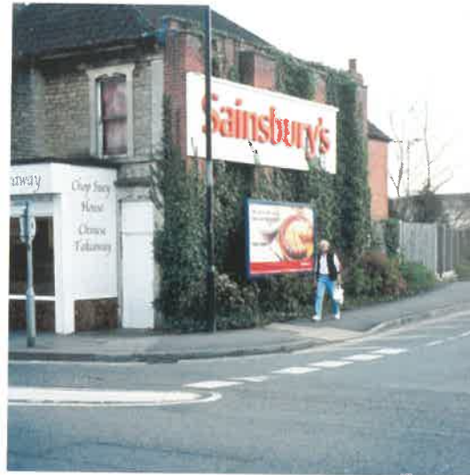
Chop Suey, 15 Bath Road. The building has been sliced off to form the supermarket entrance
