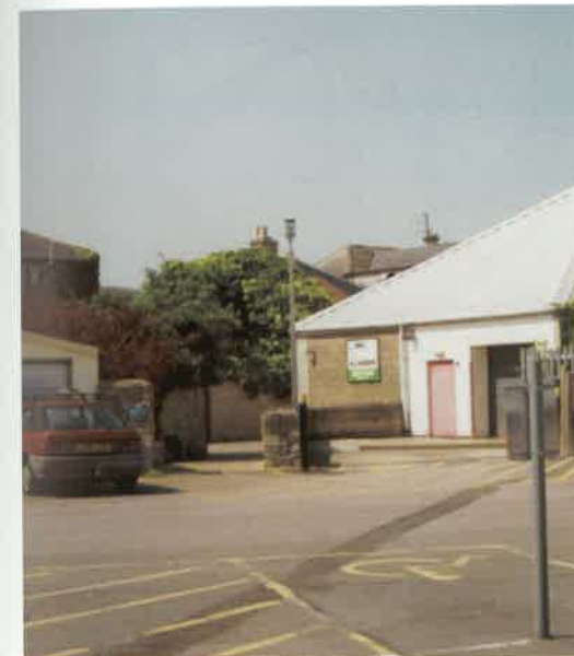
Footpath exit to King Street car park can be enhanced with a subtle design to highlight routes to shops and amenities. Project 14
