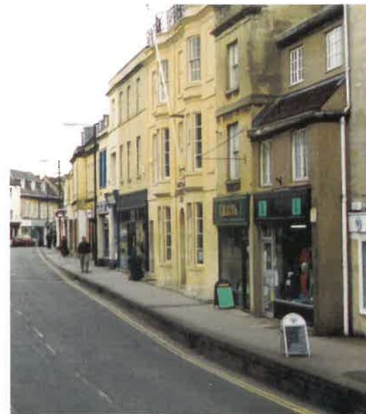
High level footpath on Bank Street is a historic feature creating a visual diversity within the street space
